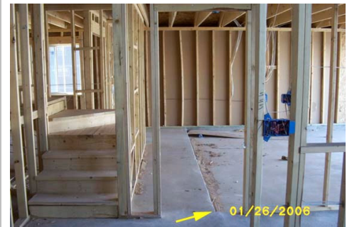
Looking @ door leading to garage – note garage step down bisects pathway in and out of door 12
