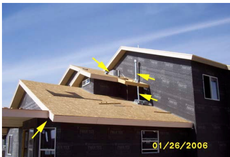
Looking @ south east corner of house – furnace and water heater flues too short and too close to vents and AC 7
